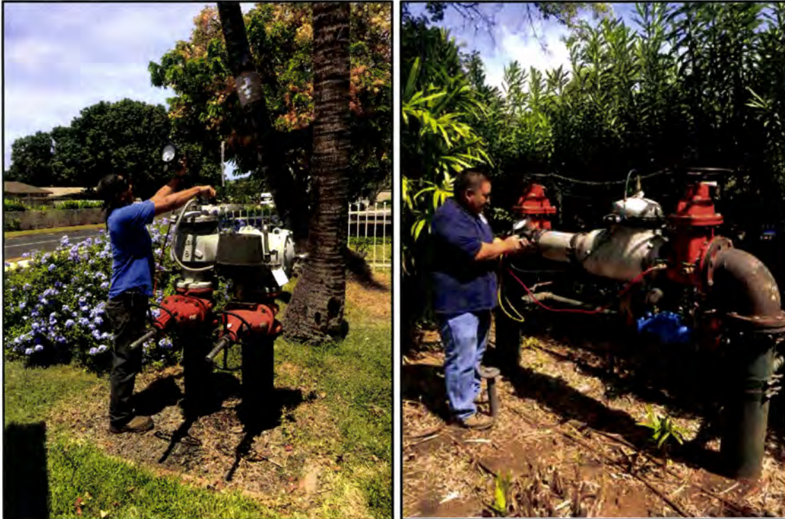
Photo Right: Back Flow Technician II Rory Honda testing a new Back Flow Preventer
